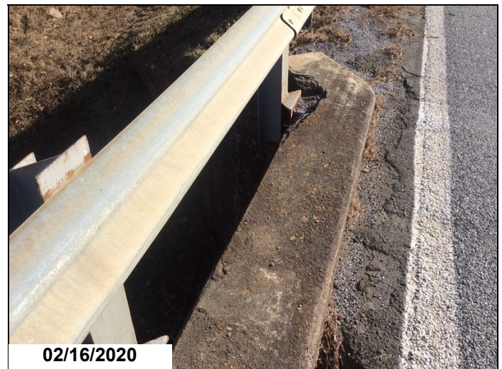
Loose bolts from impact damage
