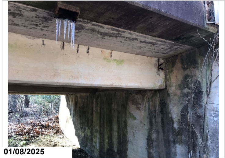
Span 1 girder 1 left side spalls with exposed rebar. CS3-7'
