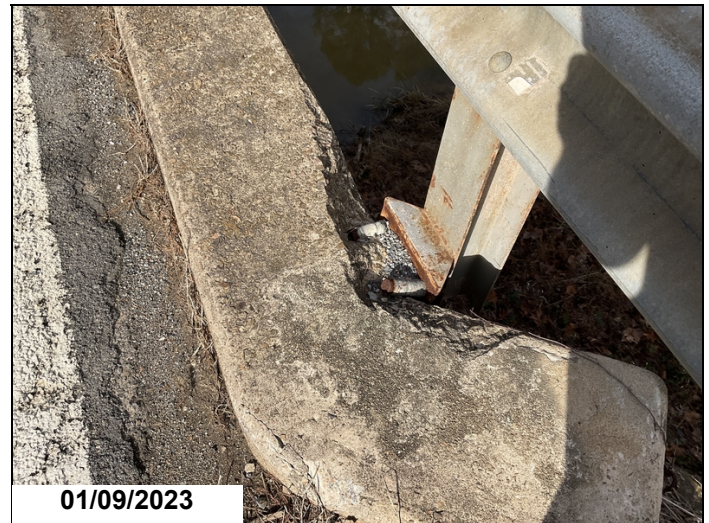
Guardrail post left side bent 3
