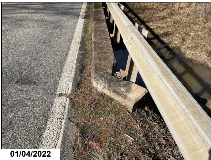
Guardrail post left side bent 3
