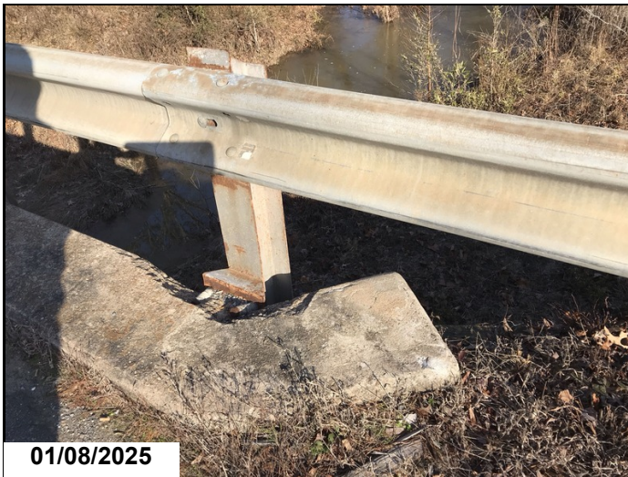
Bent 3 left side guardrail post damage.
