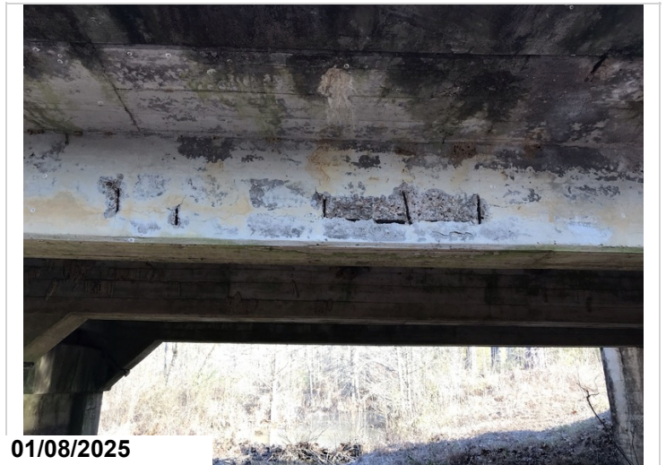
Span 2 girder 3 right side spalls with exposed rebar. CS3-4'
